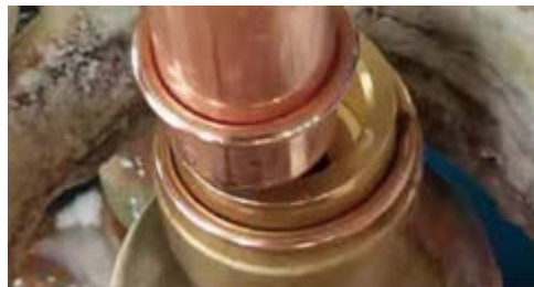
Welding of brass liquid distributor assembly
