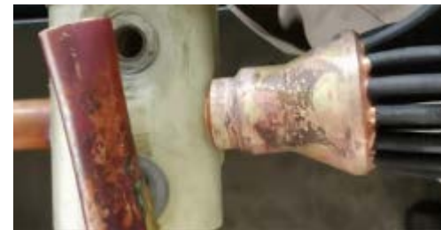
Bending and positioning distribution pipe
